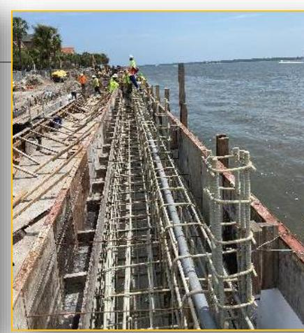
GFRP double mat for bridge deck reinforcement & pile cap
