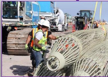
Partially prestressed 18"x18" pile using pretensioned #4 GFRP bars & auger-cast piles
